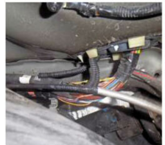
The connecting plug for the warning light wire is in a ridiculously inaccessible position.
